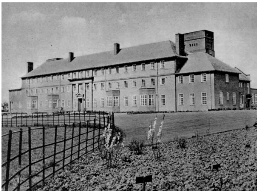
MAIN BUILDING at the Yorkshire Institute of Agriculture. The building houses 80 residential students, each of whom has his own study-bedroom.
